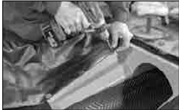
Fig 232 - Hopper transition flashing
