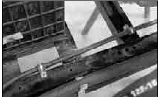
Fig 43 - Fuel hose clamped behind battery
