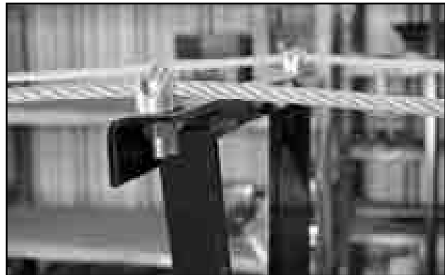
Fig 254 - Cable bridging clamps
