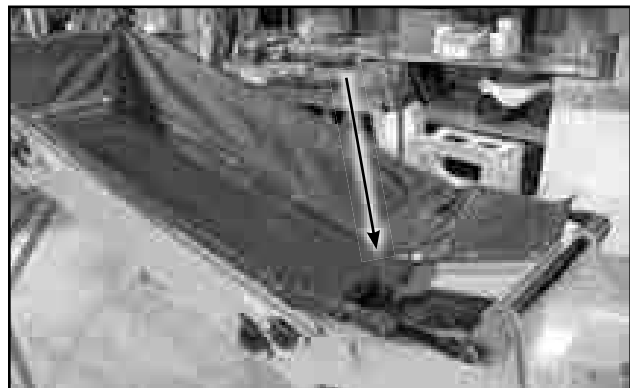
Fig 234 - Tuck corner flashing below roller
