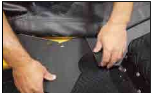
Fig 104 - Transition, Corner flashing
