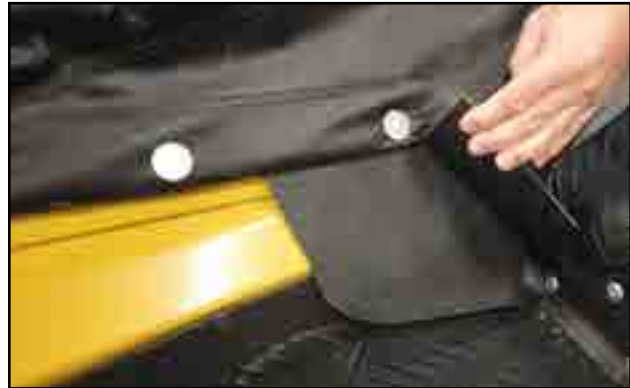
Fig 106 - Flashing fastened along transition
