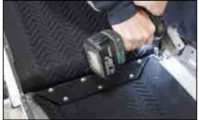
Fig 101 - Fasten transition flashing
