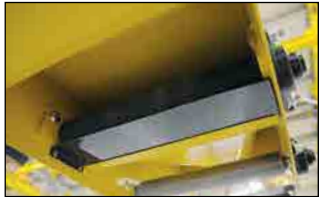
Fig 84 - Containment plate in place
