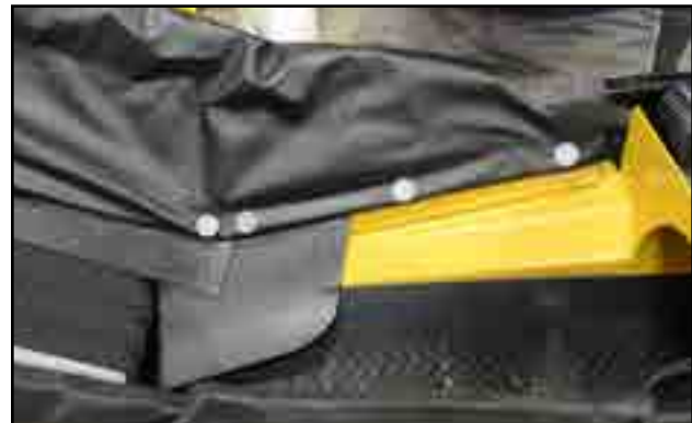
Fig 93 - Transition corner flashing in place
