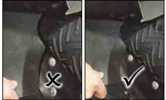
Fig 109 - Corner flashing must fit tight
