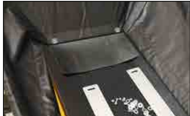
Fig 92 - Tail flashing on top of side flashing
