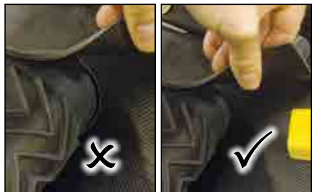
Fig 214 - Corner flashing must fit tight around the belt
