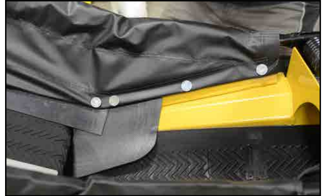
Fig 4 - Transition corner flashing in place
