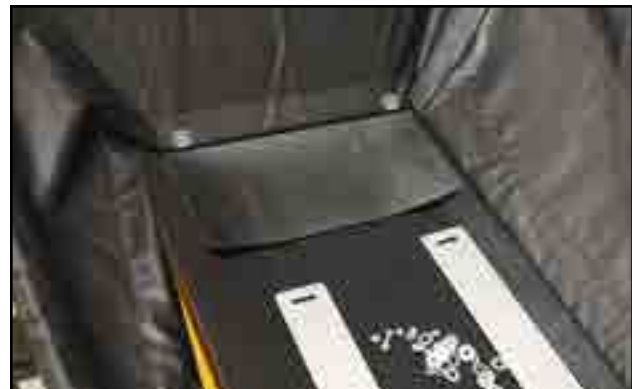
Fig 111 - Tail flashing on top of side flashing
