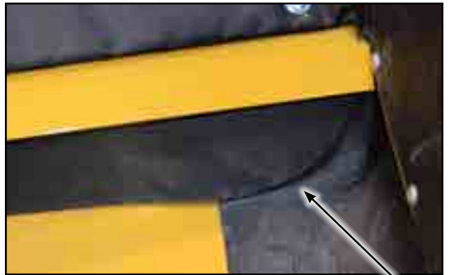
Fig 108 - New side flashing
