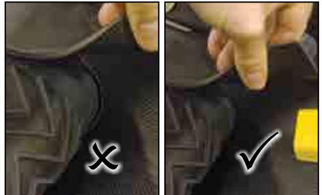
Fig 114 - Corner flashing must fit tight around the belt
