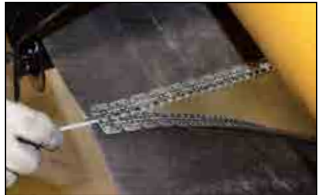
Fig 101 - Thread lacing cable
