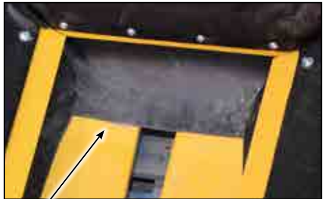
Fig 107 - New tail flashing
